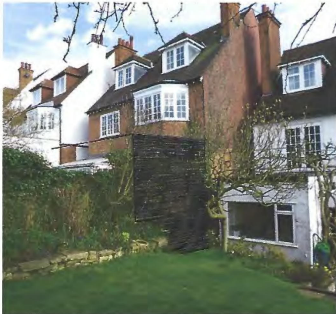
Fig 2 photo from garden of 29 Crediton Hill, showing relative elevation of 29 and 31. Area shaded is where extension's flank wall will be.
