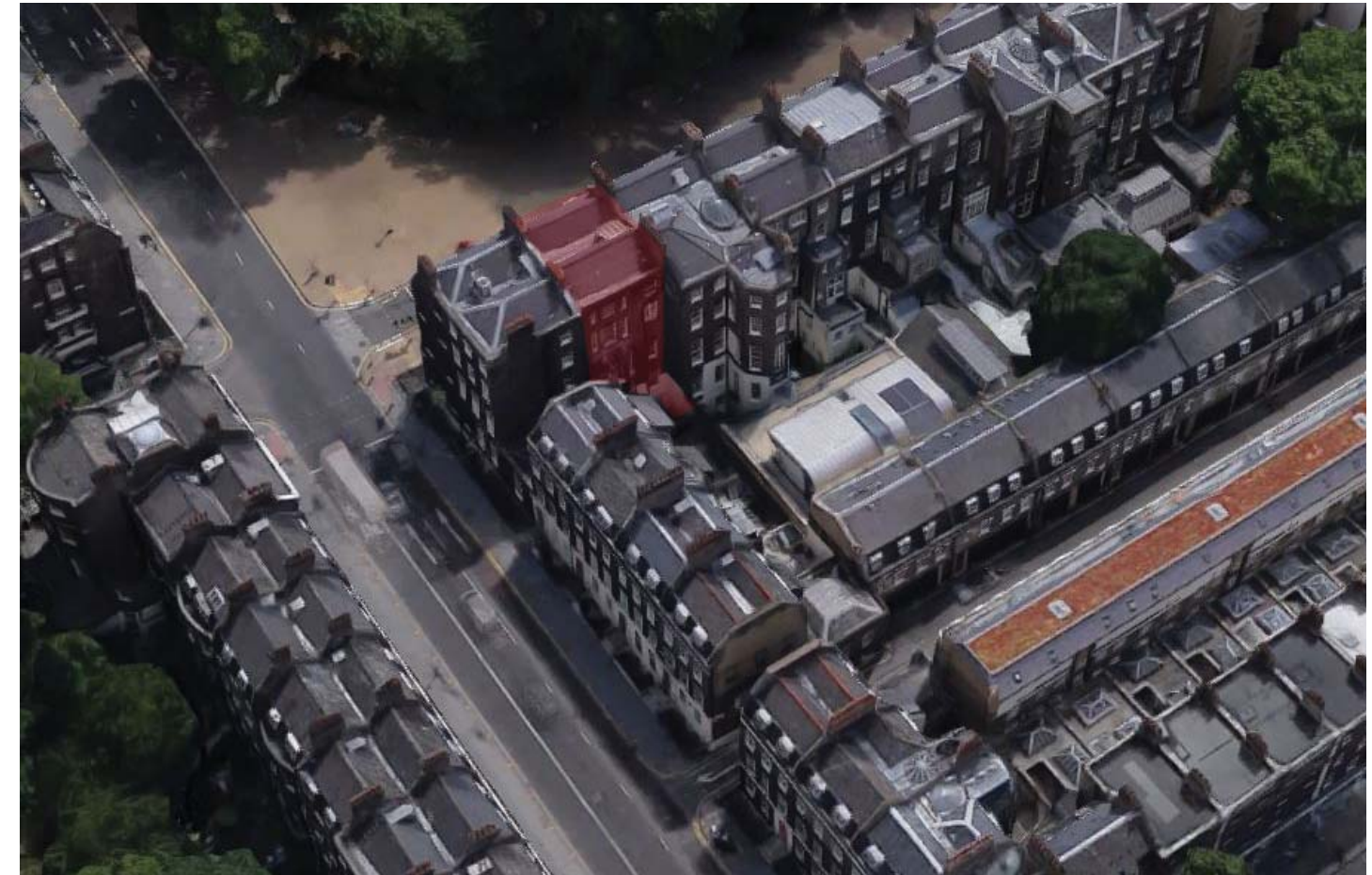
Aerial View of 13 Bedford Square from the North
