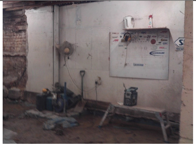
View north of basement
