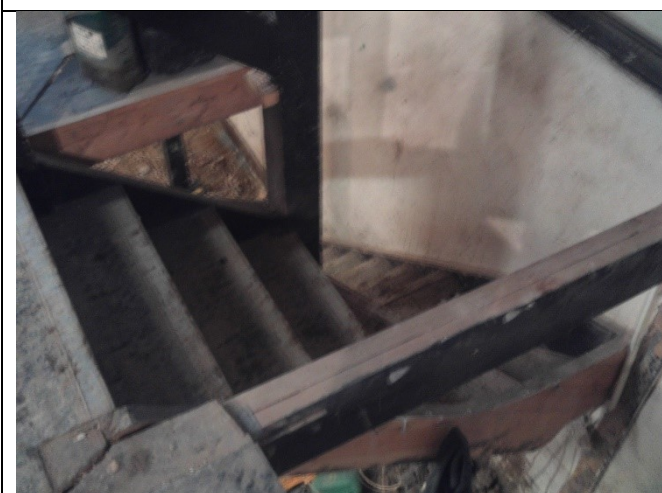
View of stairs leading to basement
