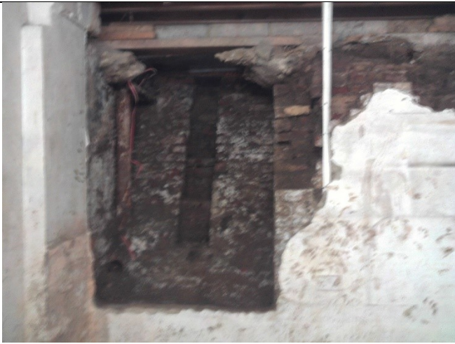
View north-east of basement
