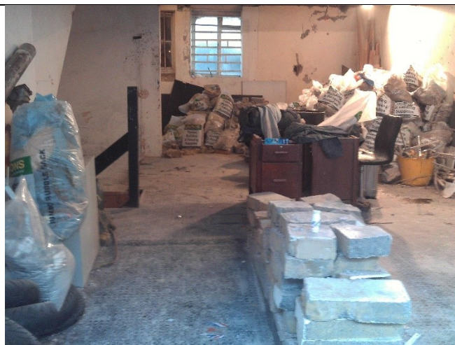
View from site entrance to the rear of the site
