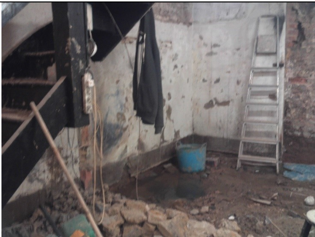
View south of basement
