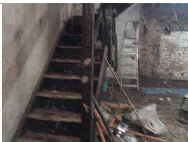
View of basement stairs leading to ground floor
