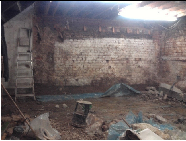
View east of basement
