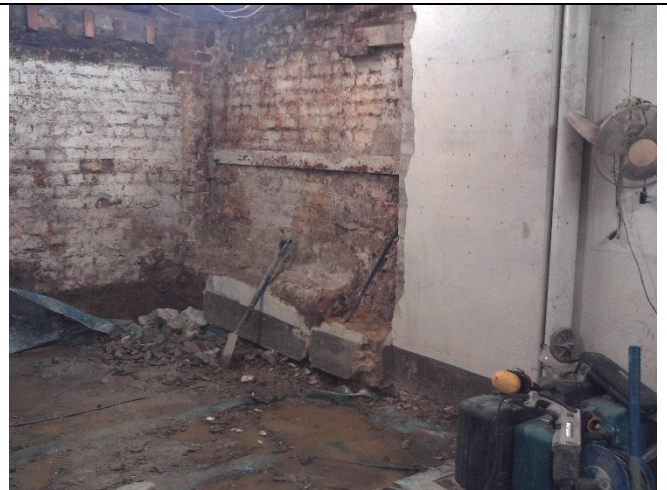
View north-west corner of basement
