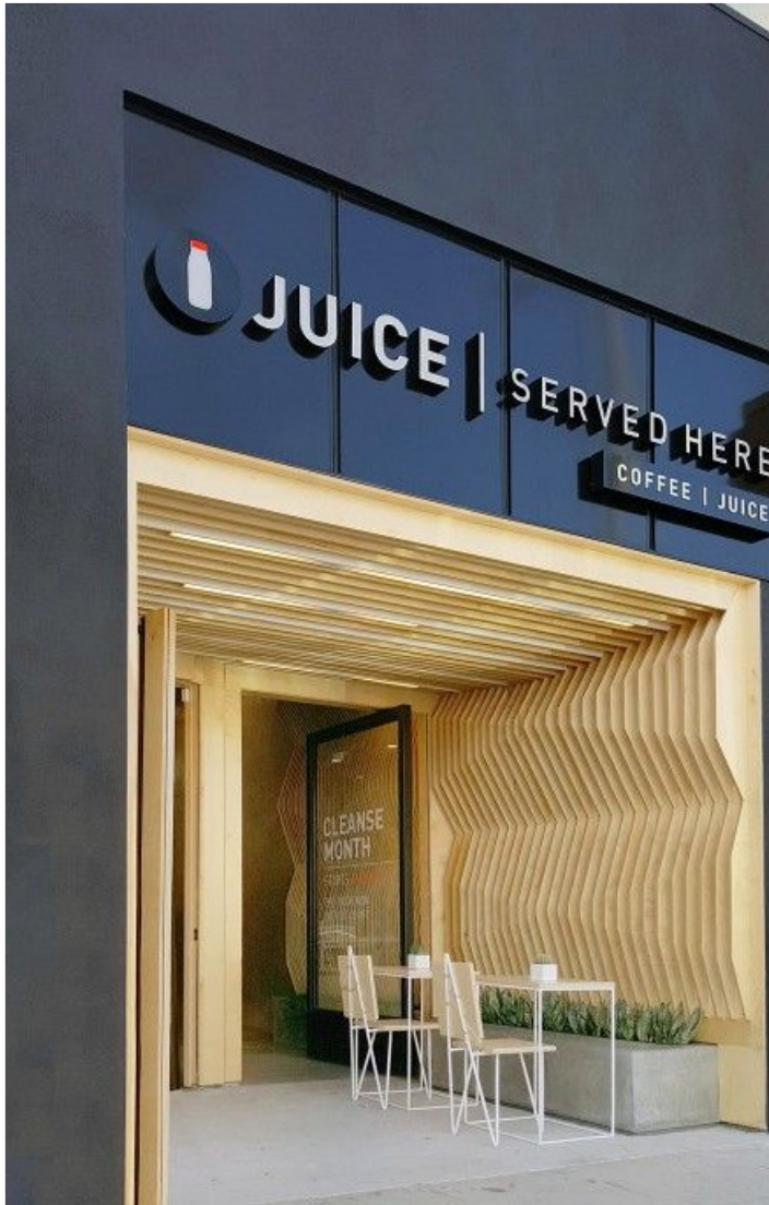
Proposal for cladding for external entrance – dark grey cladding panels to cover green stone, timber from reception within reveal to create continuity between inside/outside spaces.
