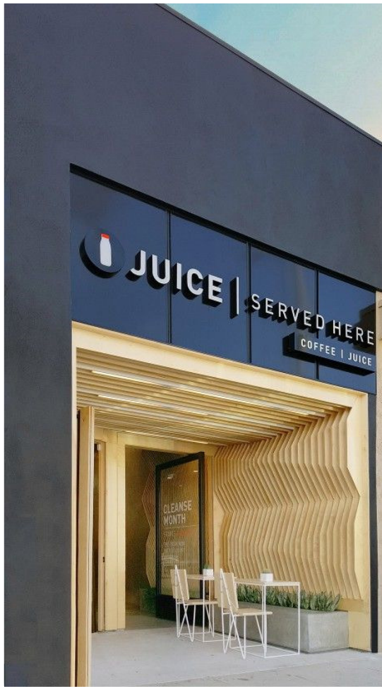
Fibre cement panels alongside timber plank external cladding
