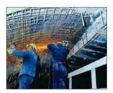
In the Brachbach tunnel project, **DELTA**\*-**PT** was installed over a quickdrying shotcrete levelling layer to provide full-surface drainage. The inward-facing mesh provided a secure bed for application of the inner shotcrete shell.
