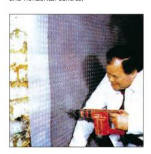
The transparent sheet allows easy location of fixings so that the brick or stone can be identified from the mortar joints. Ventilation gaps can be used at floor and ceiling level to ensure the optimum air circulation.
