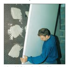
When dab fixing plasterboard the adhesive dabs are applied directly over the fixing heads. The adhesive dabs should cover 50% of the area. The boards are then wedged at the bottom and offered up to the dabs.
