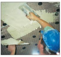
Plasters and renders should be trowel applied in two coats. The first coat is pushed into the dimples, and giving cover over the mesh of 6mm. This is lightly scratched and allowed to dry before the second coat of 9mm is applied. Skim finish plaster can be used in the normal way.
