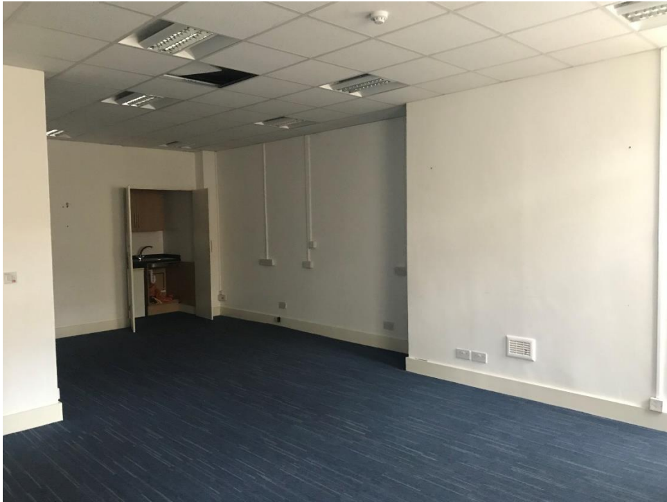
Plate 2: Basement level front room, March 2019
