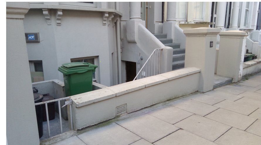
○ No.52 AINGER ROAD EXISTING CONDITION (1) NTS
