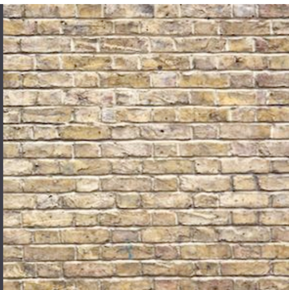
Existing walls London Stock Brick
