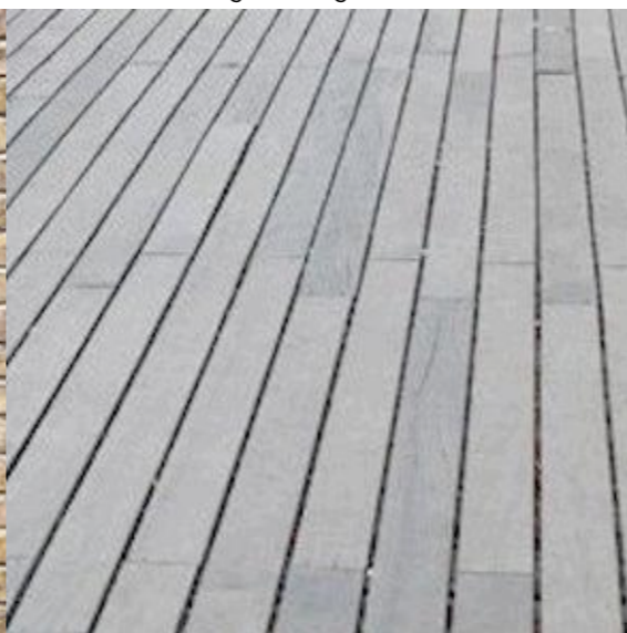
Terrace decking, internal cladding and terrace built-in furniture Plain cut Scotlarch 100mm wide planks with copper screw fixings
