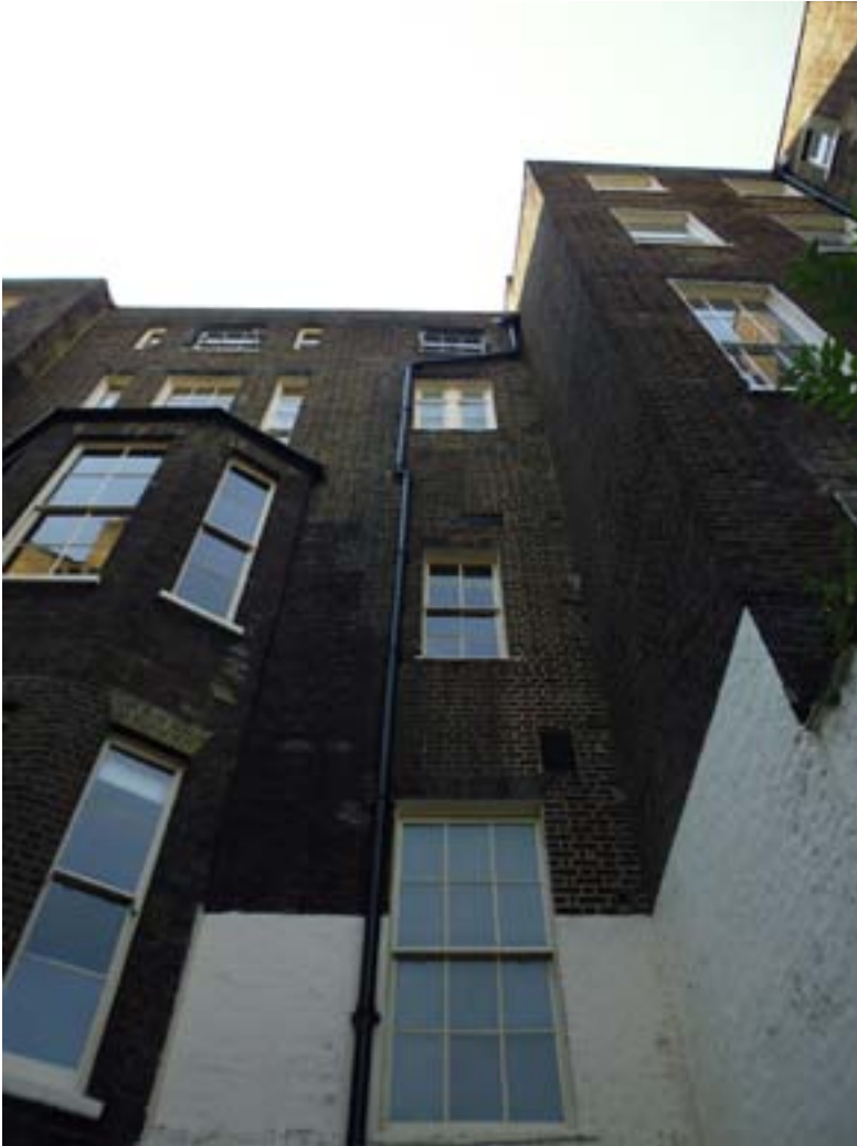
Photograph of Rear Elevation showing evidence of existing openings
