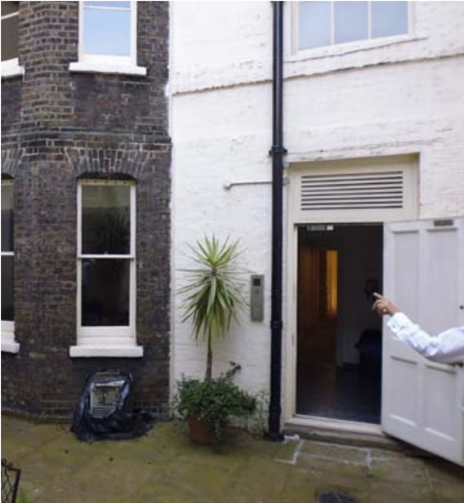
Photograph of Rear Elevation at Lower Ground Floor Level
