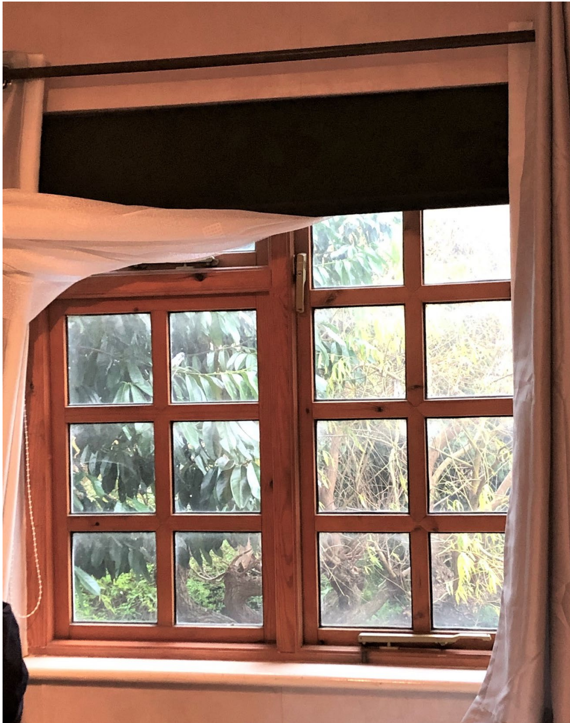
Figure 8: Internal view of window at first floor bedroom (Flat 4)
