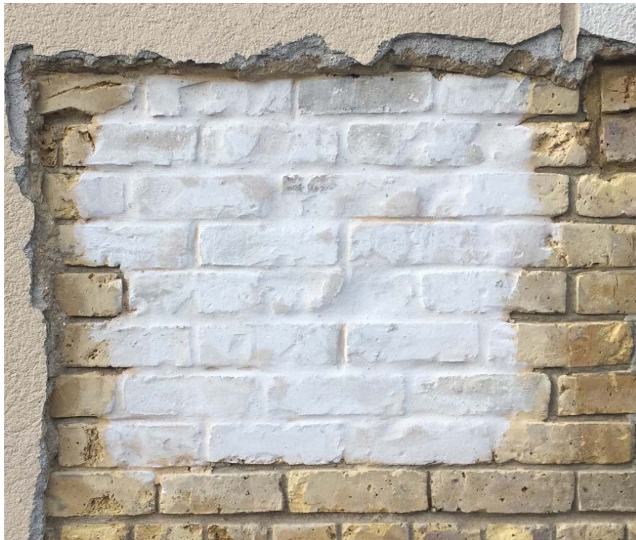
Plate 5: Overview of brickwork following repair and 1 tinted coat of Keim Restauro
