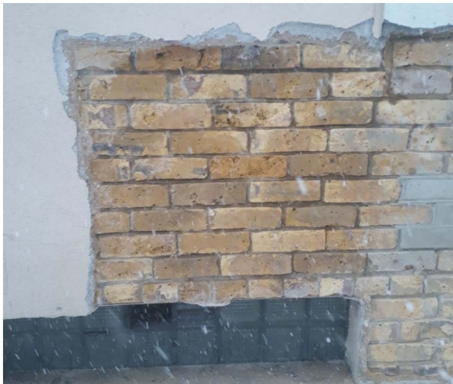
Plate 2: Area following completion of render removal
