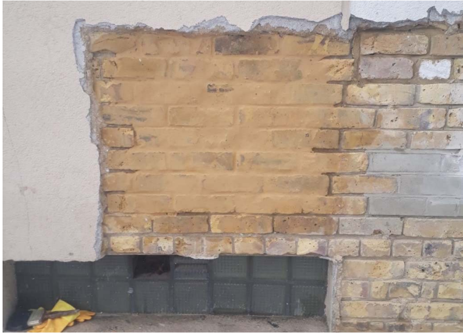
Plate 3: Area following repair and repointing
