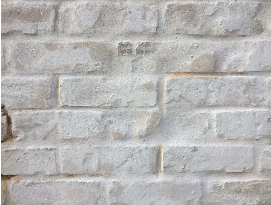
Plate 6: Detail of brickwork following repair and 1 tinted coat of Keim Restauro
