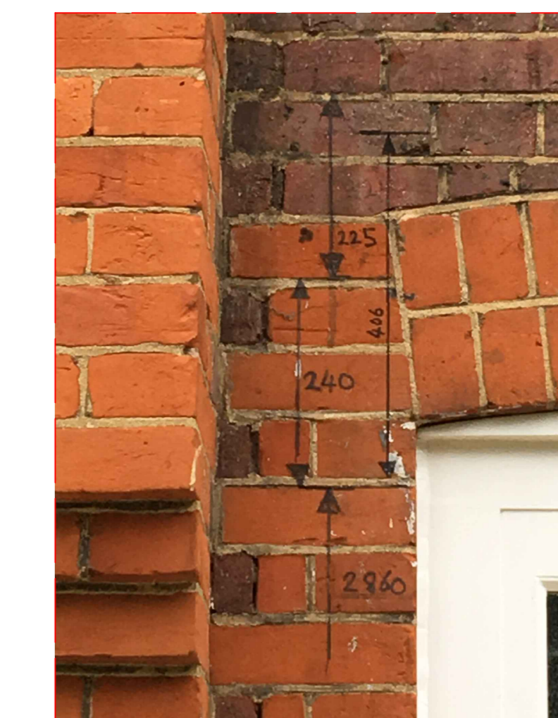
CONTRAST BRICKWORK DETAIL New brickwork to match
