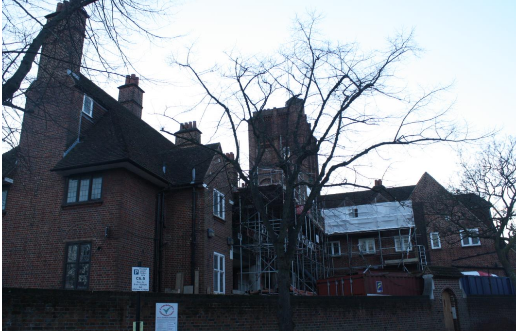
CONSTRUCTION WORKS IN PROGRESS ON SITE
