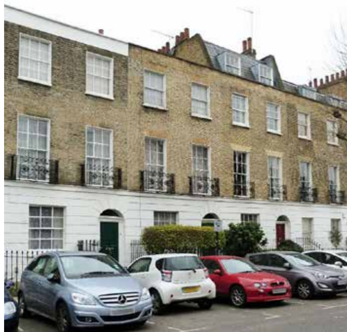
EXISTING BUILDING, FRONT VIEW
