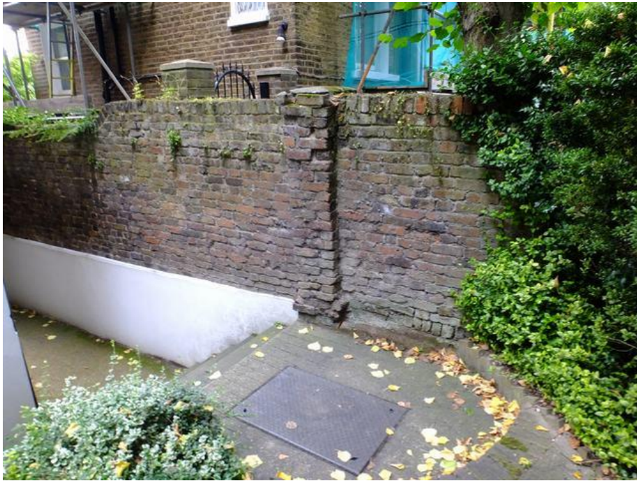
Image 11 Inspection cover for existing services, so roots likely to have been restricted or severed
