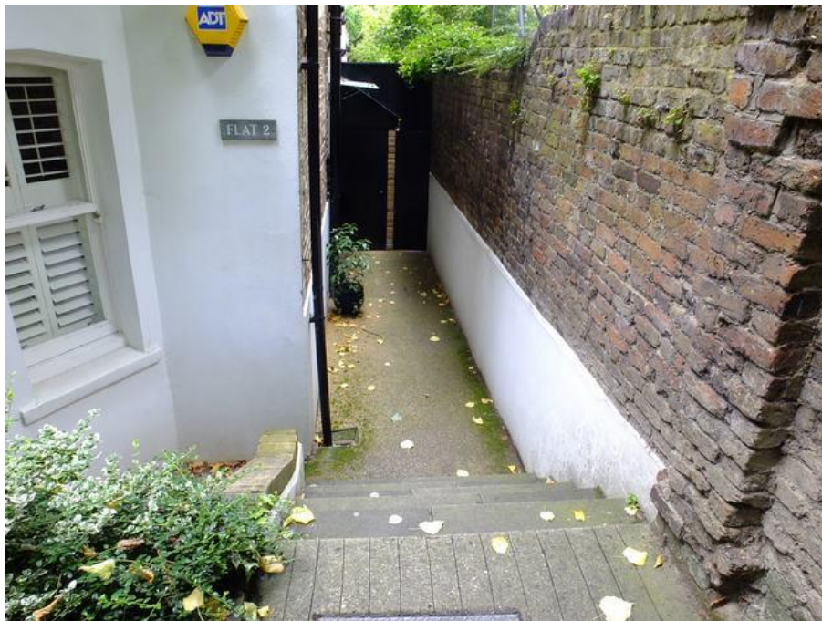
Image 12 Steps leading down to the entrance, with some space for materials
