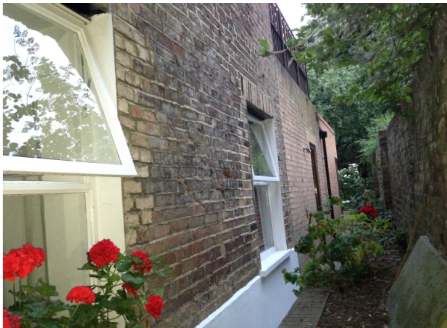
Fig 2 - Rear of side passage way (behind existing boiler shed)
