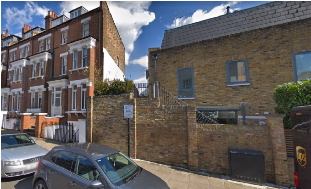
2) Stairs leading to terrace with existing visible balustrade and planting
