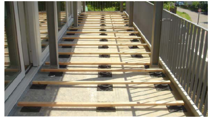
under structure for wood decking
