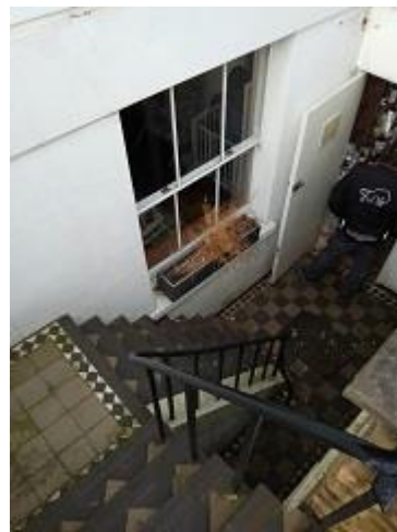
Access to Vaults
