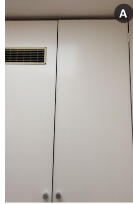
Boiler Cupboard Asbestos lined boiler cupboard recently removed following an asbestos survey.
