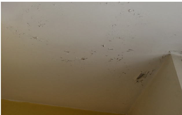
Bedroom 1 En-suite - Ceiling
