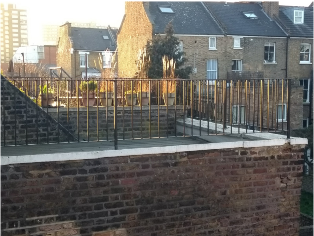
Proposed railings to be 750mm high from parapet level
