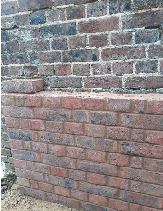
Sample wall (different mortar, existing wall in behind)
