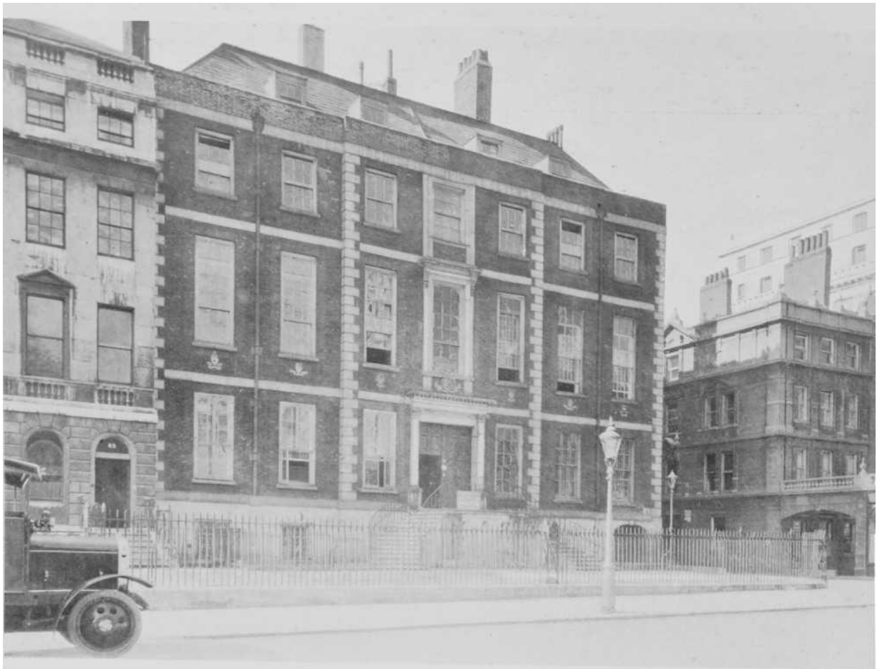
Figure 22. Powis House, 1924. Note development of central bay of the main façade including division of entrance steps and the loss of the central pediment.
