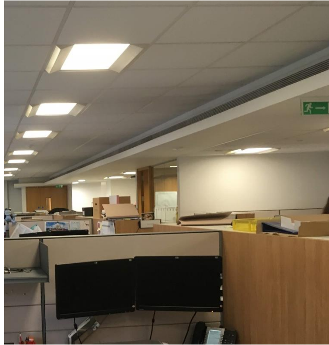
Figure 14. Late twentieth century standardised office layout to the interior with suspended ceilings, strip lighting and secondary glazing throughout. These areas are without interest.
