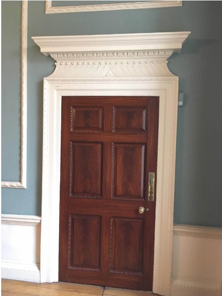
Figure 25. Decorative plaster moulding to interior, indicative of eighteenth century design.
