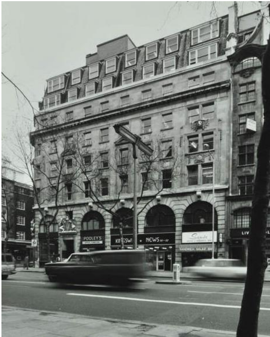
Figure 9. Street photography of the site 1978, viewed from Kingsway to the west. Note plant work to roof, visible in this image.
