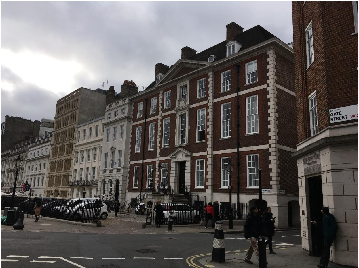
Figure 11. View south along the western boundary of Lincoln's Inn Fields. Note variety to the facades along the terrace as seen to the left wall as the blank character of the side façade of Powis House to the right, creating a formal hierarchy to the elevations. Note the location of the proposed works is not visible in this image.
