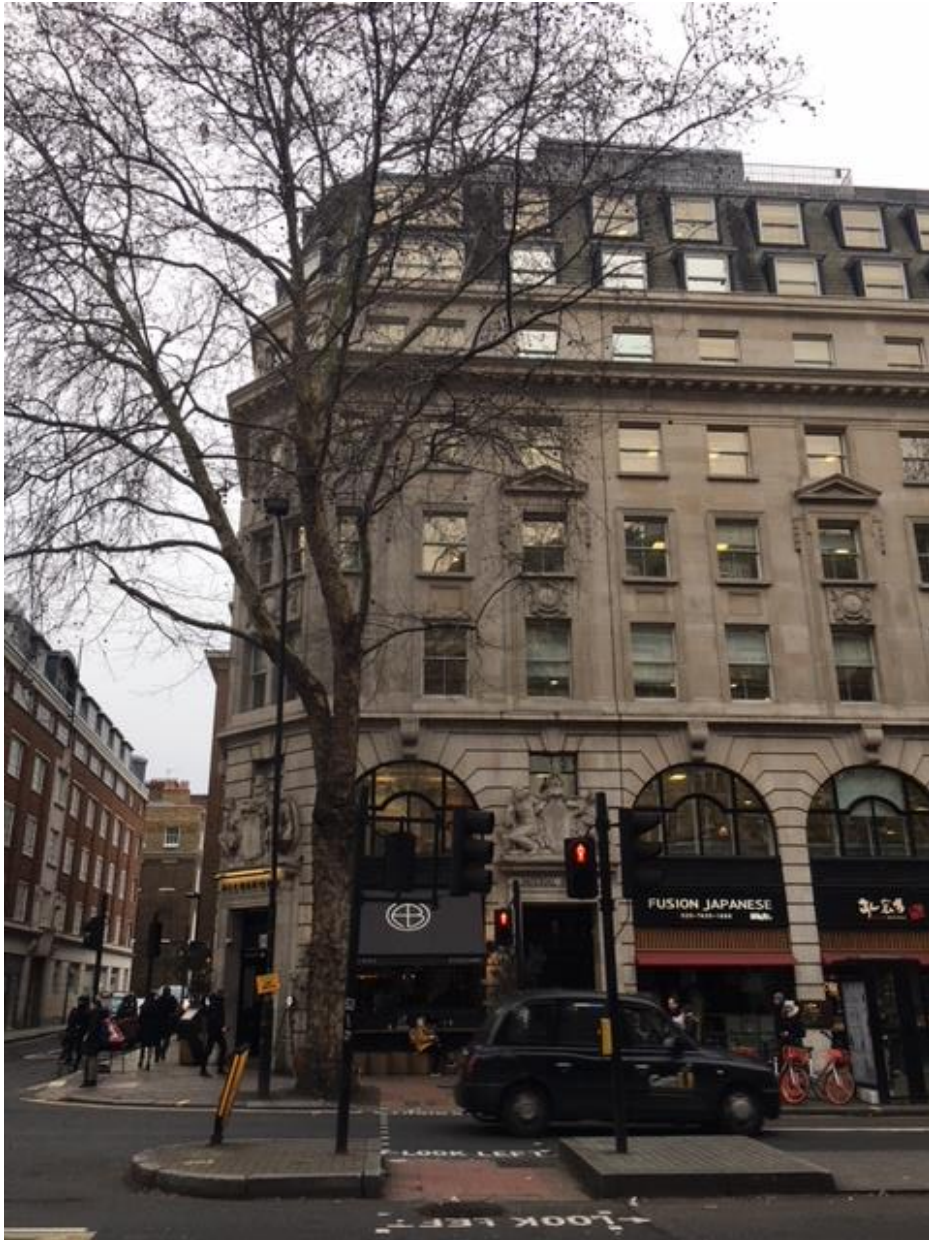
Figure 12. View of Imperial Buildings seen from Kingsway to the west. Note view of existing screen to roof seen at street level, as well as the contrasting massing, scale, decorative character, materials and aesthetic of Imperial Buildings when compared to Powis House.
