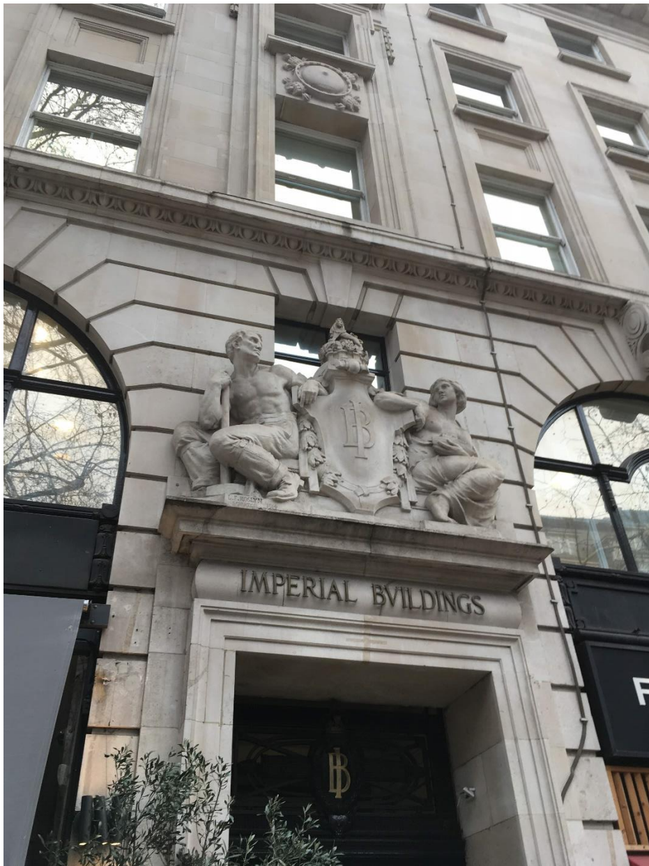
Figure 13. Decorative sculpture over entrance to Imperial Buildings. Note rustication of ground floor and use of Portland Stone facing to the facades.
