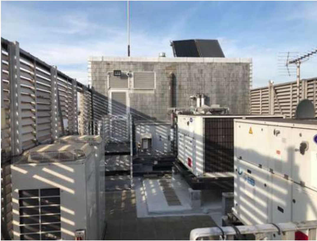
Figure 1. Location of the existing units, to be replaced, looking north.
