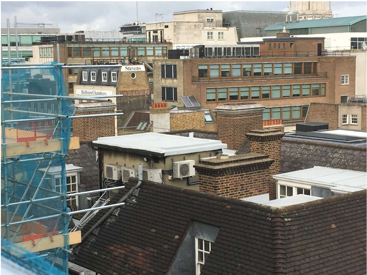
Figure 5. View of plant work within the surrounding roofscape.
