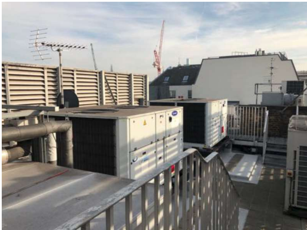
Figure 2. Existing units to be replaced, looking south east.
