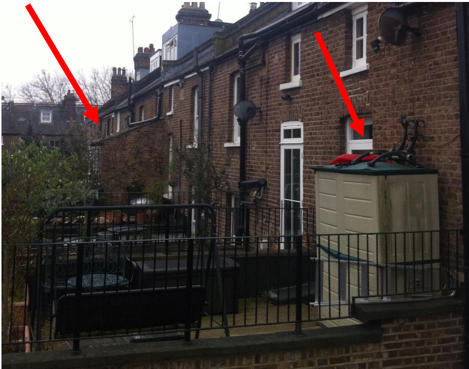
Above: Rear additions on neighbouring properties terraces as viewed from the application site
