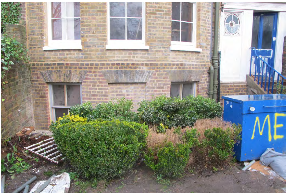
Fig. 4.2A Rear of house showing basement lightwell
