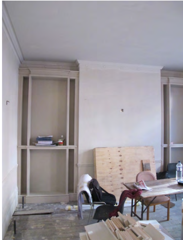
Fig. 2.2A Over-boarded ceiling, pre-2017 works
