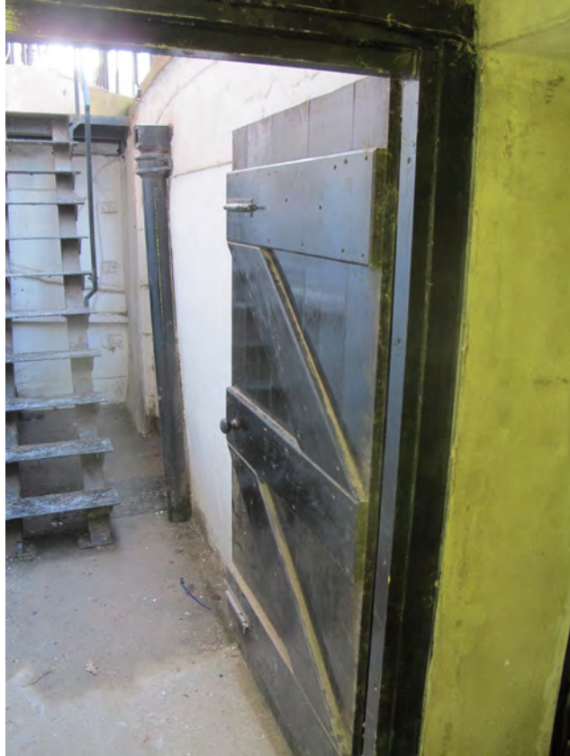
Fig. 3.1B Existing basement entrance door, internal view
