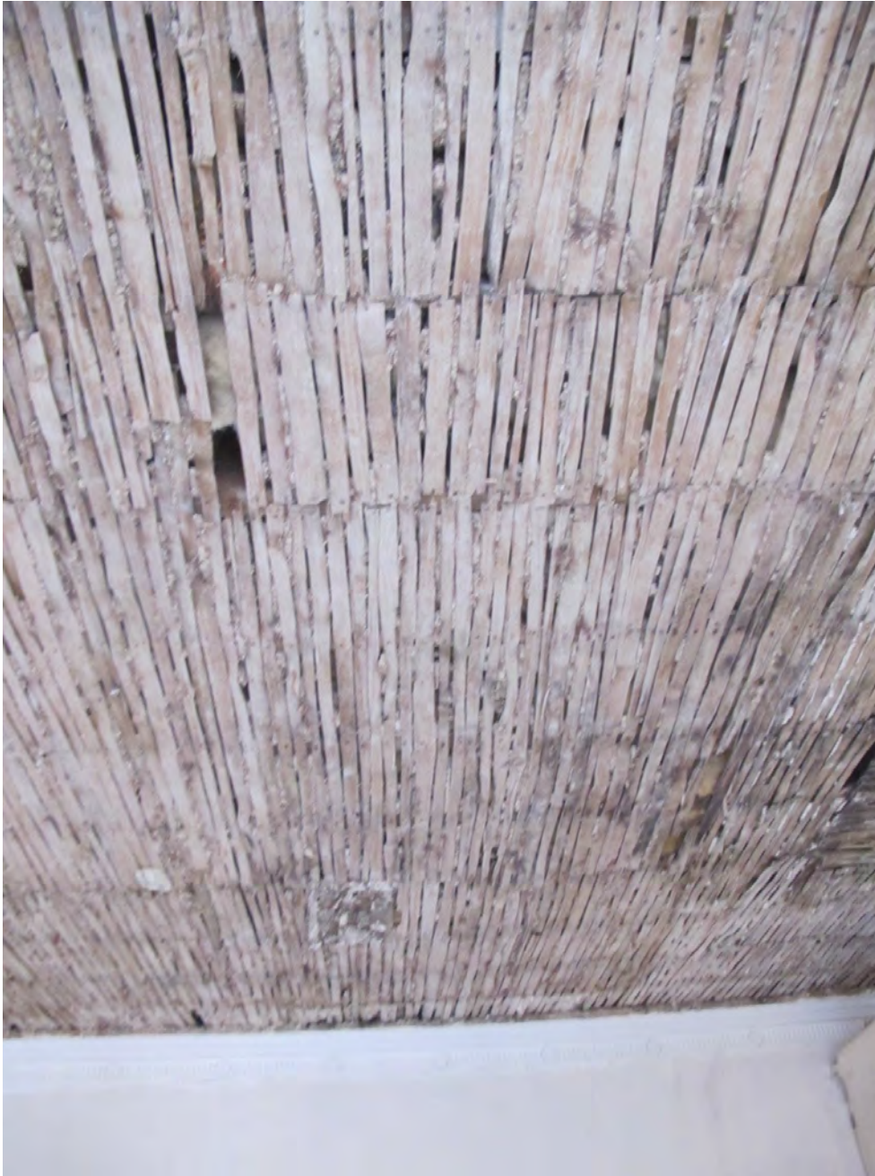
Fig. 2.2E Lathing with loose lime plaster removed
