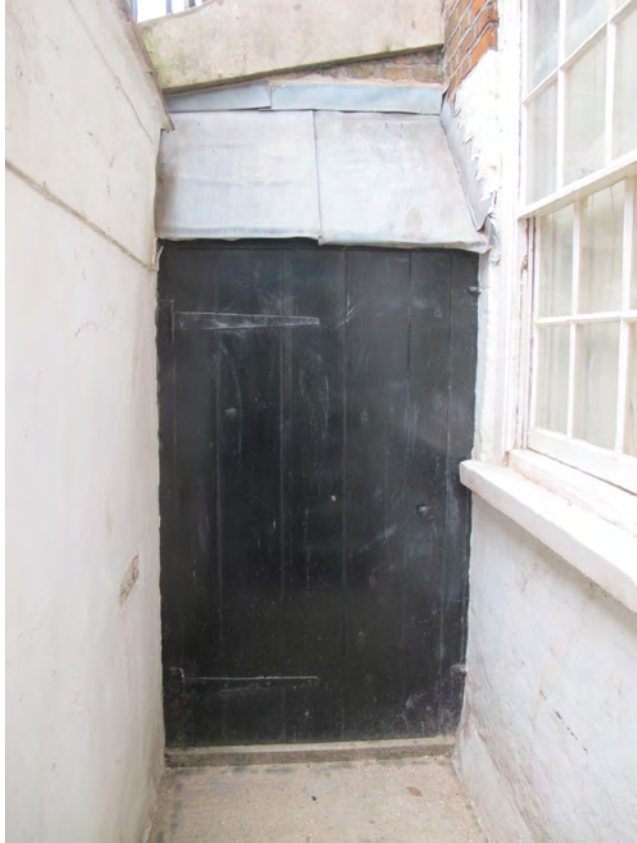
Fig. 3.1A Existing basement entrance door, external view
