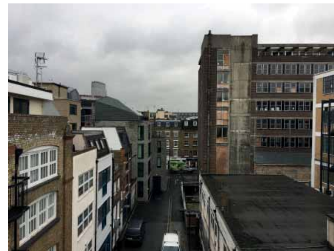
View down Tottenham Mews from Roof of 13 Tottenham Mews
