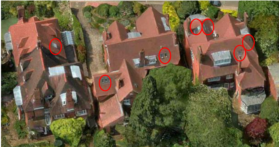
Nos. 48, 46, 44 to the south
