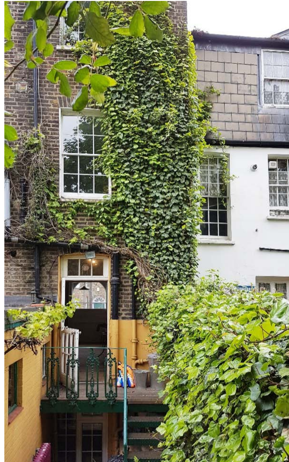
Existing rear elevation of no.133 showing the lower ground windows covered by stairs and decking
