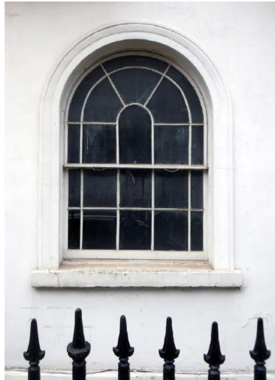
Front Elevation - Historic arched sash window and external render
