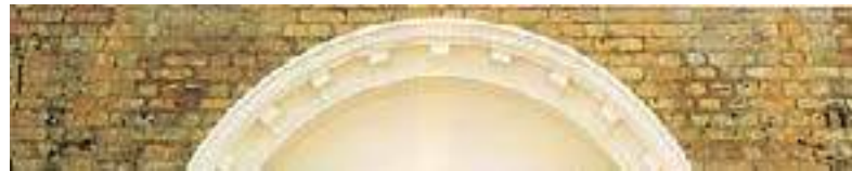
An example of the type of stains which may appear on a 'cleaned' facade if inappropriate methods or procedures of cleaning are applied.
