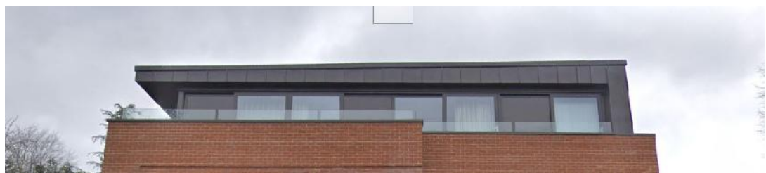
Fig. 2 Roofing at 38 Redington Road: Vertical standing seam metal panels clad the second storey
