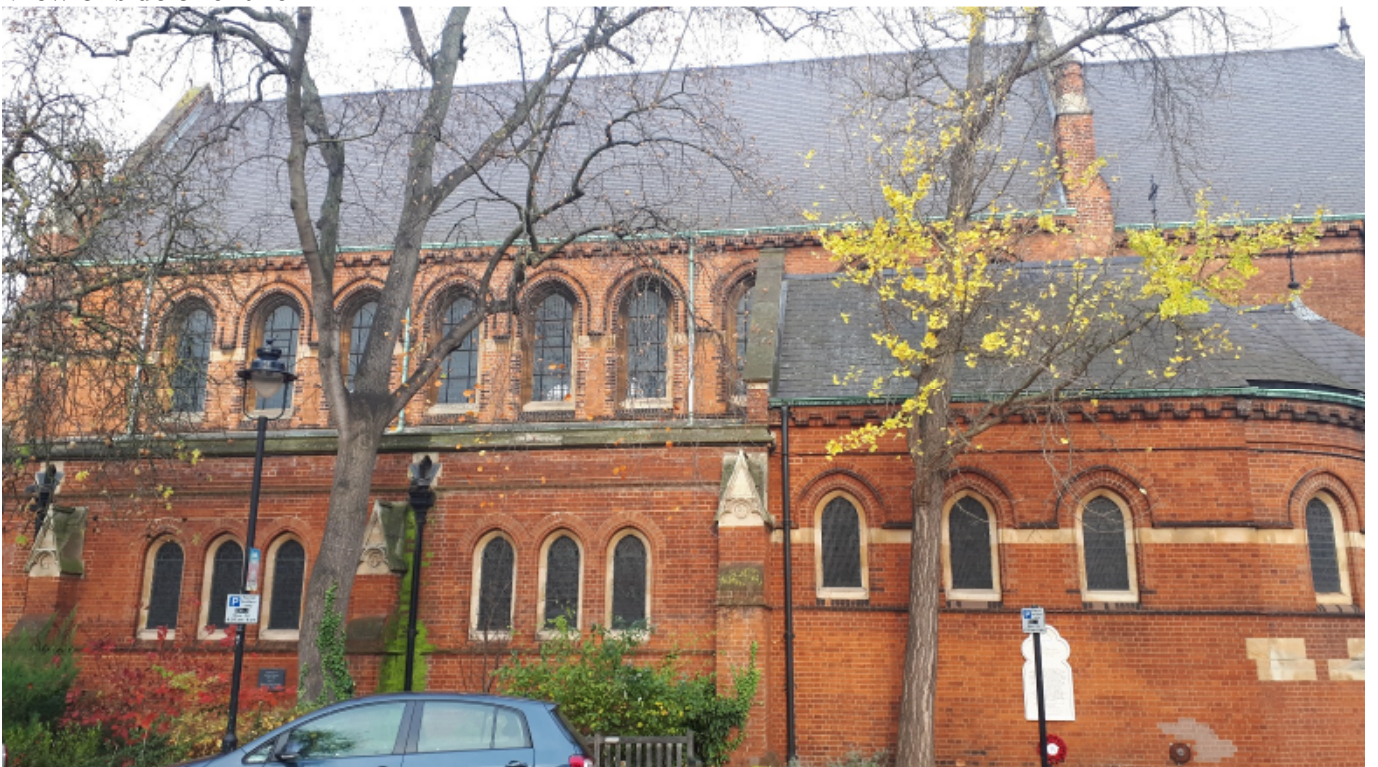
View of side of church
