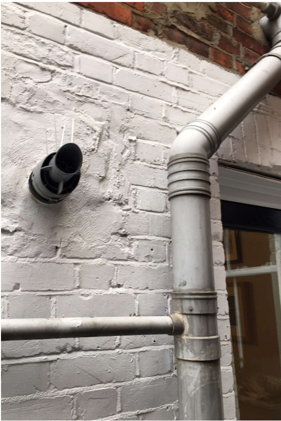
Poor quality white painted brickwork to rear and side walls to be improved. Pipework to side wall to be rationalised
