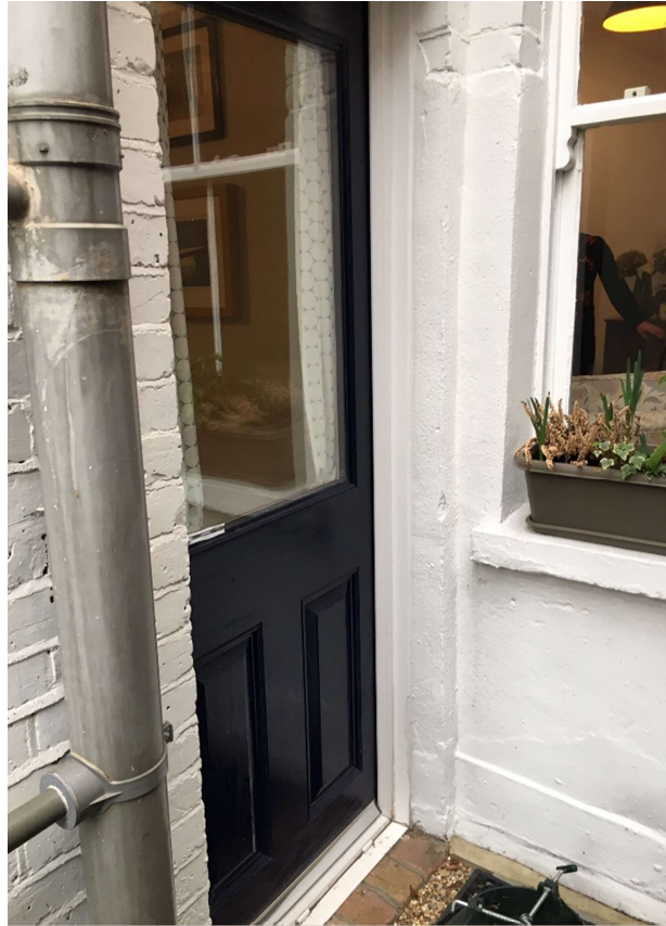
Poor quality white painted brickwork to rear and side walls to be improved. Pipework to side wall to be rationalised
