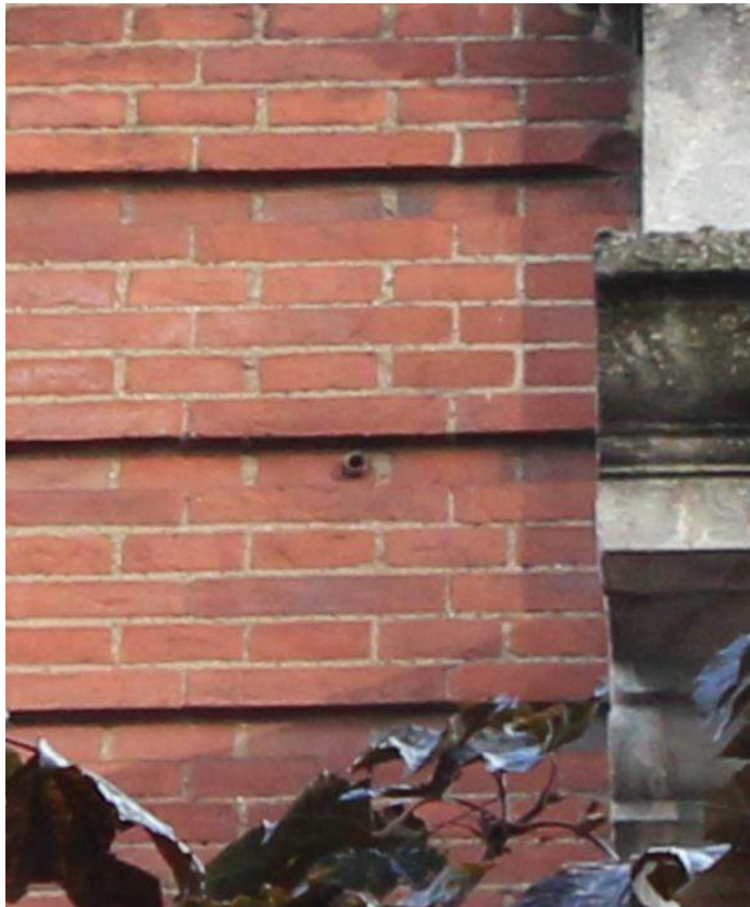
Figure 4: An existing scaffold tie in the masonry
