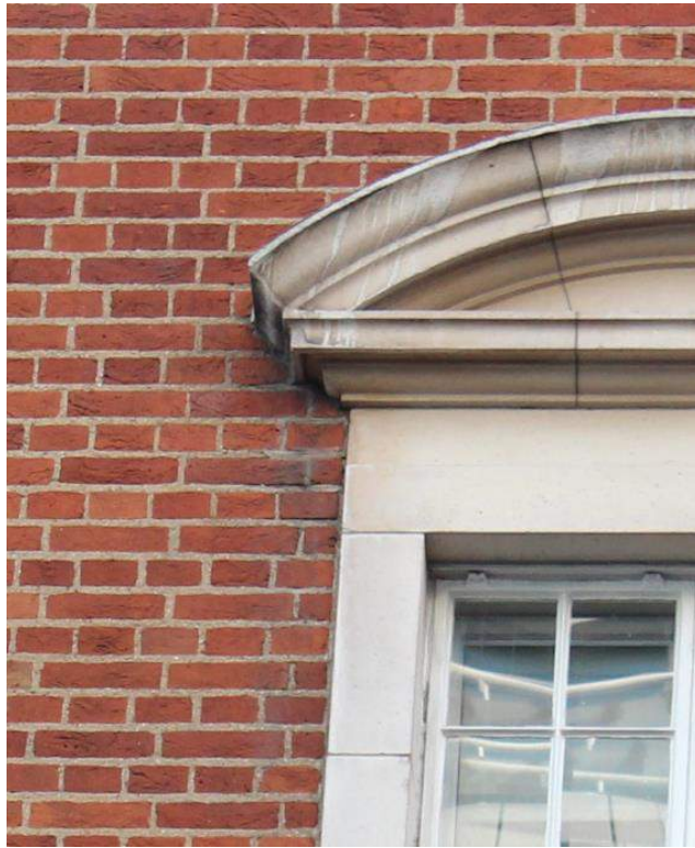
Figure 3: Water damage down the side of the windows
