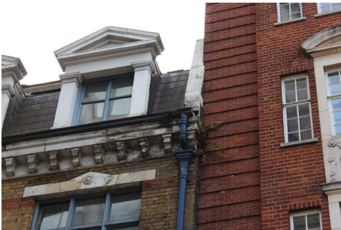
Figure 5: Evidence the downpipe has previously been blocked, with vegetation growing
