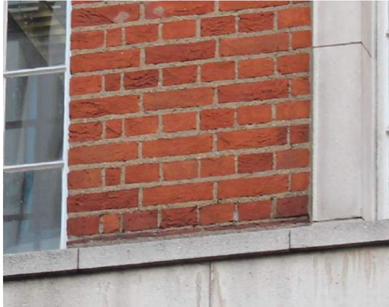
Figure 2: Evidence of damage to the mortar above the sill
