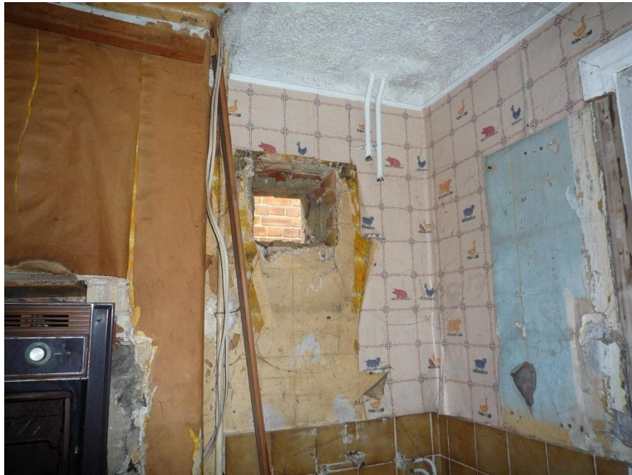
Picture 3 – House 1, large open vent in kitchen
