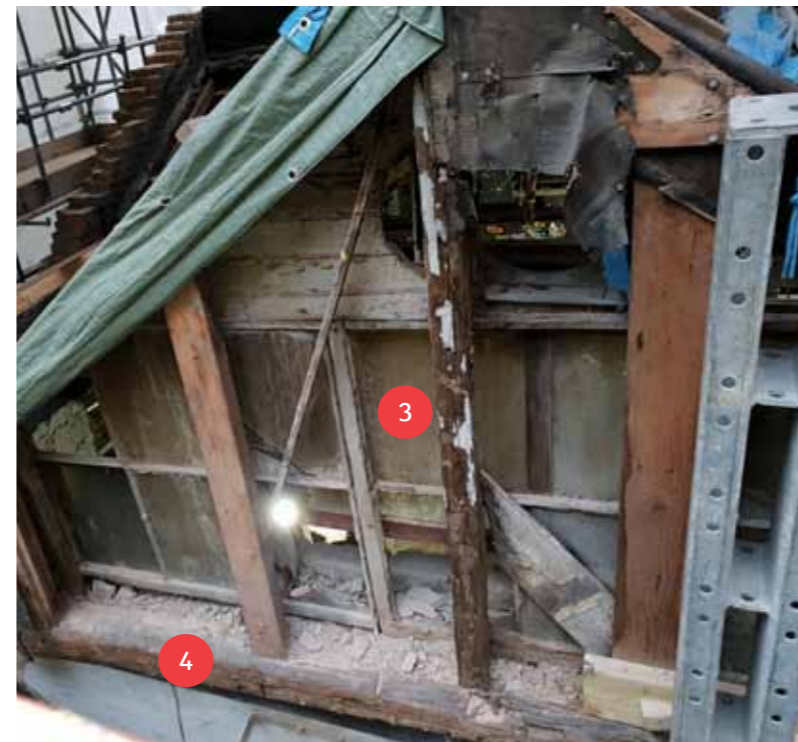
Photographic record following removal of existing felt tiles
