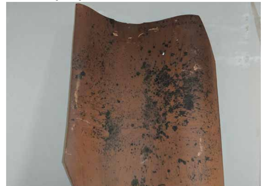
Photo of Existing Tiles (Following removal of roof coating)
