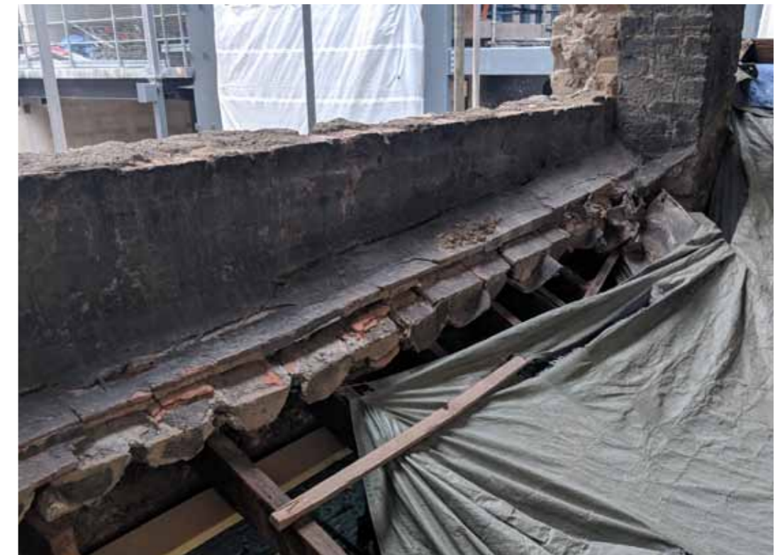
Photo of remaining existing tiles
