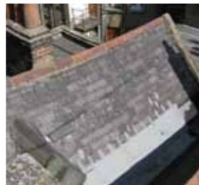
Reference image: 26 Denmark Street Roof
