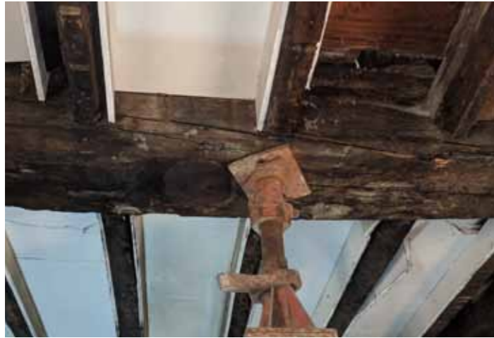
1 Existing spine beam at first floor
