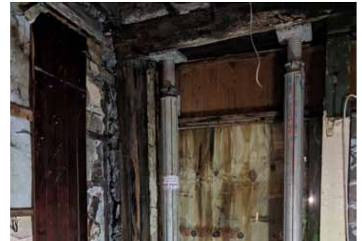
5 Existing bessemer beam support
