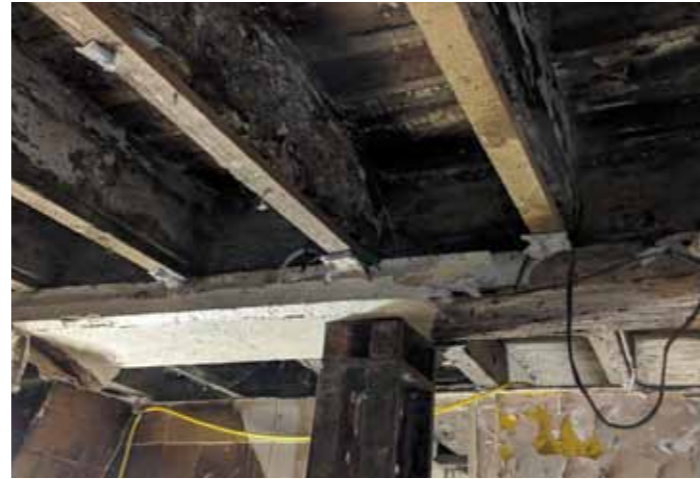
1 Existing spine beam at lower ground
