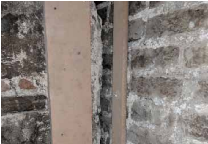
3 Existing chimney independent from party wall
