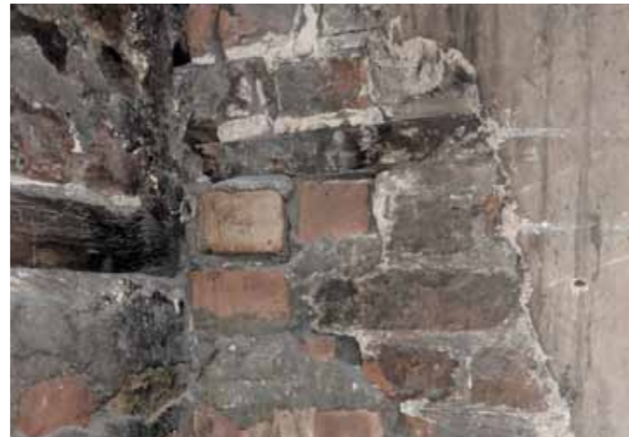
4 Existing masonry corner
