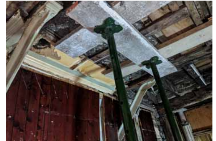
3 Existing chimney support
