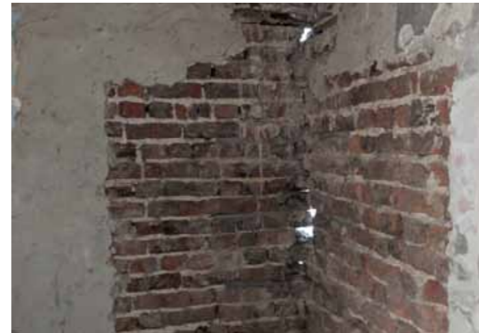
4 Existing masonry corner
