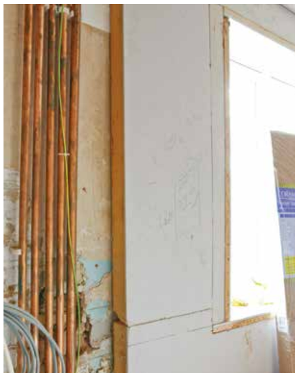
Detailing was particularly important around window reveals and access to services.
