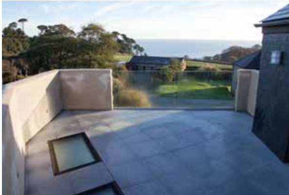
Kingspan OPTIM-R™ Balcony & Terrace System installed on the new terrace.
