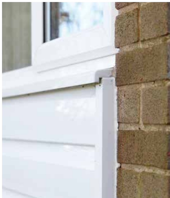
Kingspan OPTIM-R™ External Wall System was installed behind the u-PVC facade.
