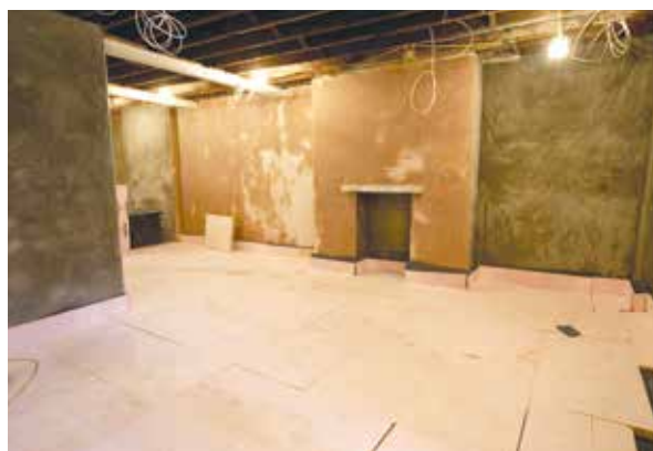
Kingspan Kooltherm ® K3 Floorboard, installed in the basement.
