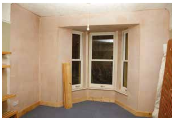
Internal wall insulation used in the front room on the front elevation.
