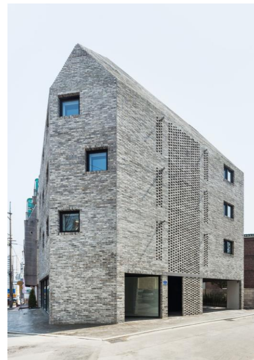
3. PERFORATED SINGLE BRICK WALL FOR OUTDOOR CIRCULATION
