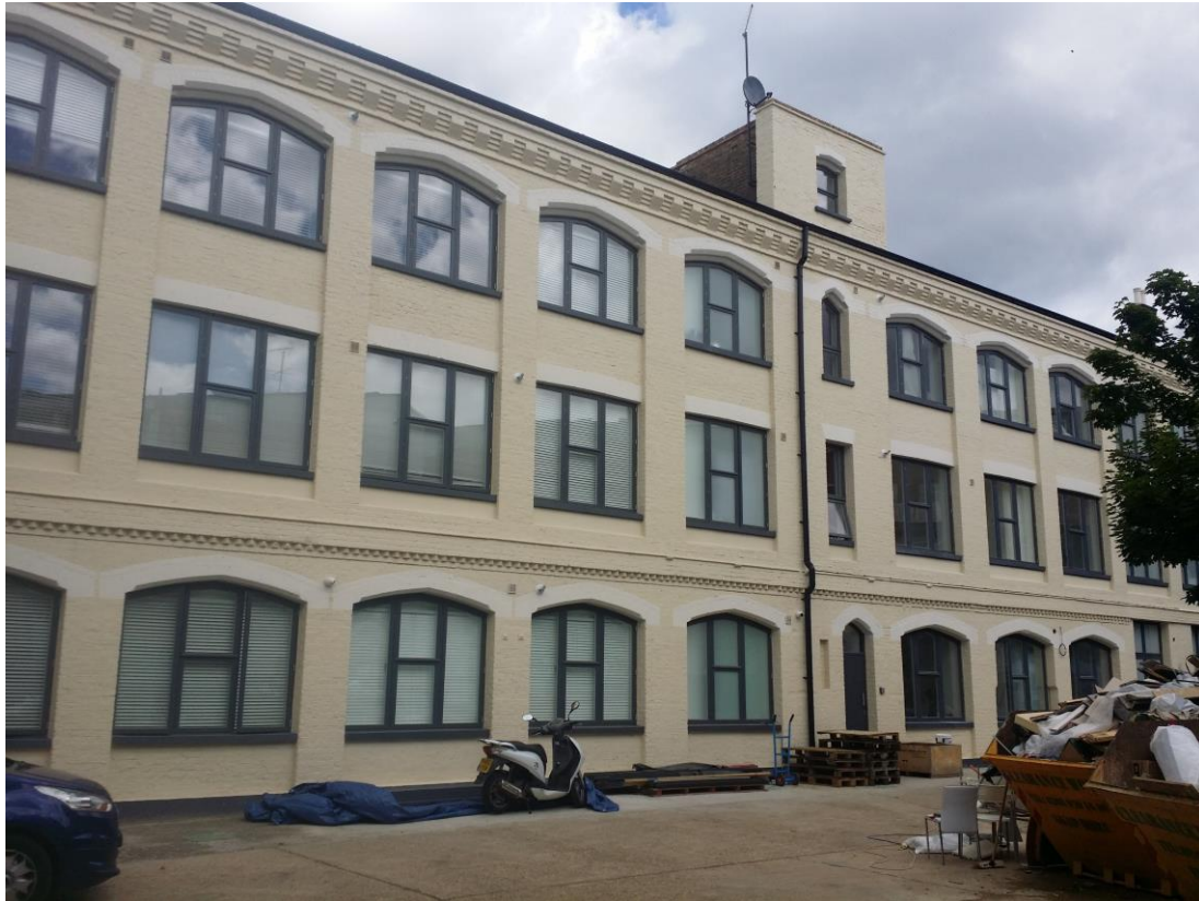
REAR 5-8 ANGLERS LANE, NEIGHBOURING PROPERTY, BRICK PAINTED OFF-WHITE
