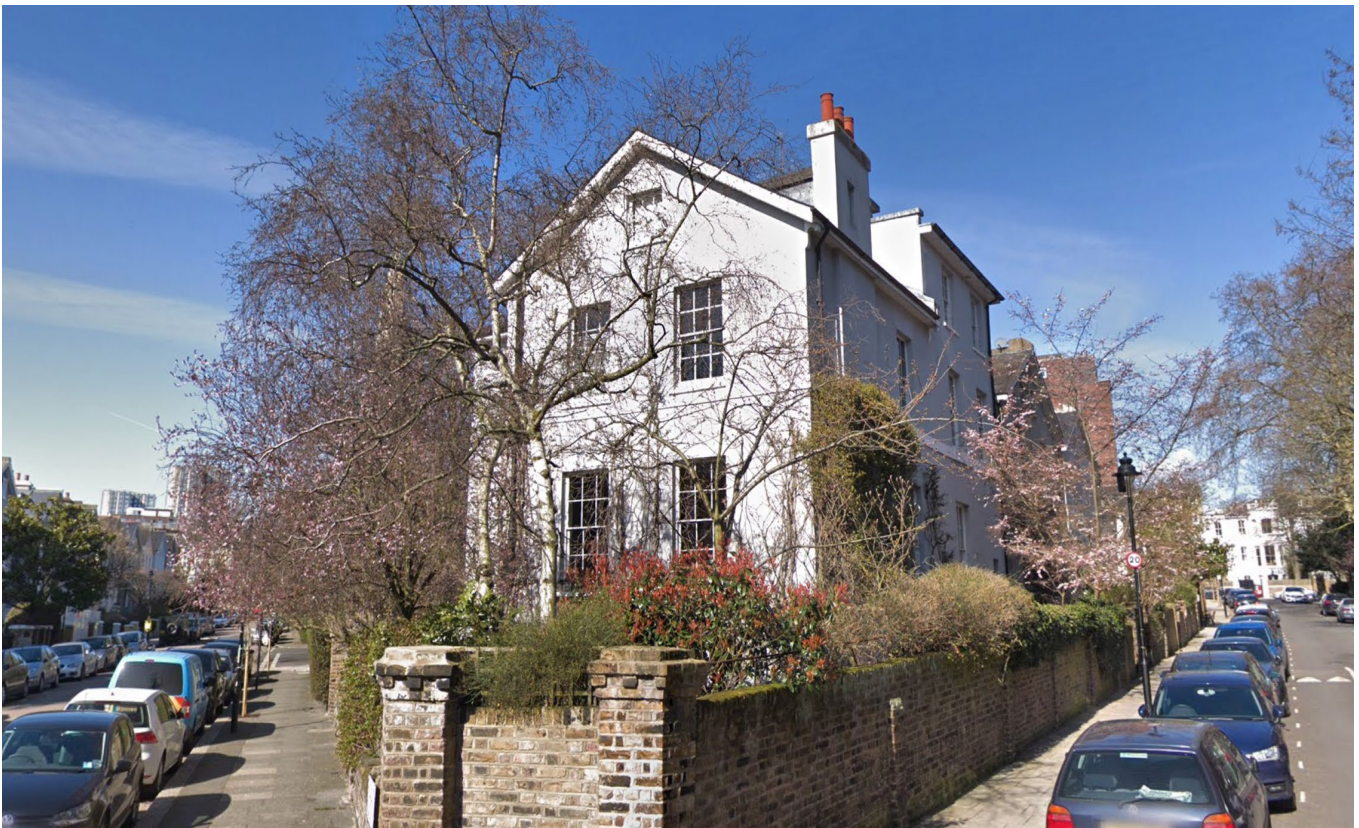
Fig 3.0 - South Elevation of 1 Eton Villas
