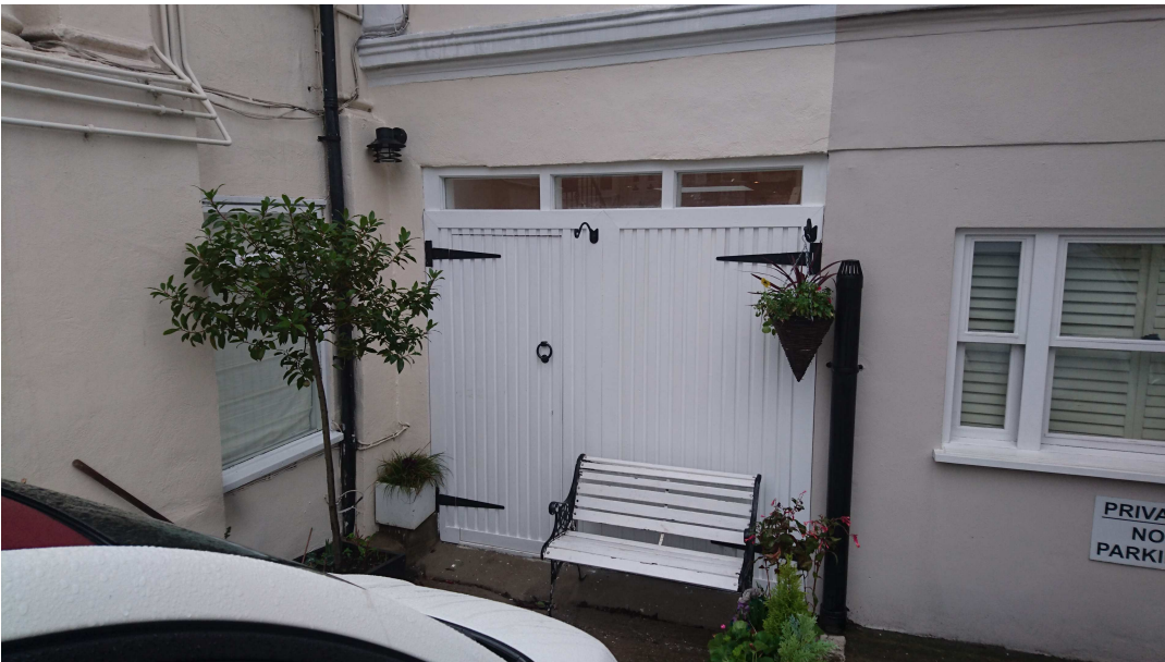
Existing door set
