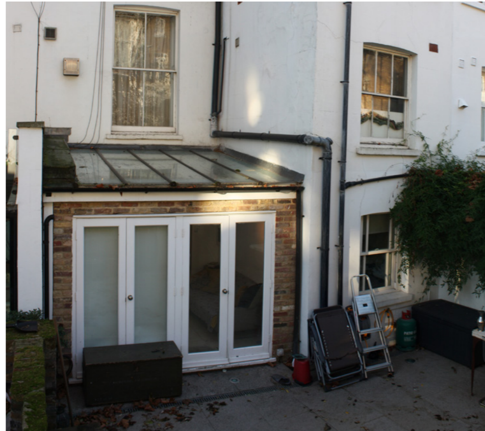
View of the existing rear extension
