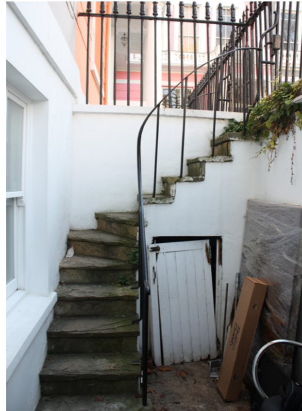
Entrance stair from lightwell
