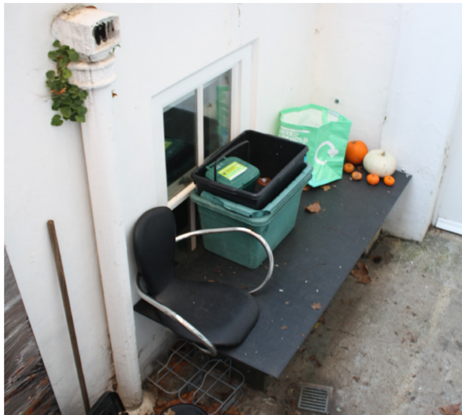
Vault window to lightwell
