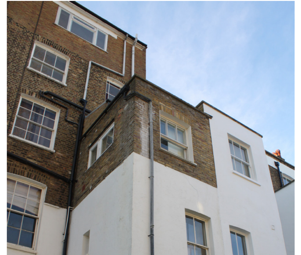
View of the closet wing
