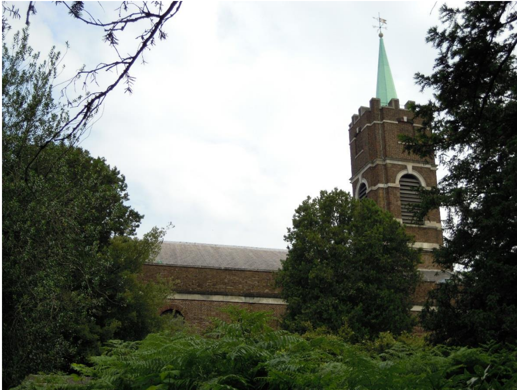
3. View of south facing nave roof from clearing in churchyard (July 2018)
