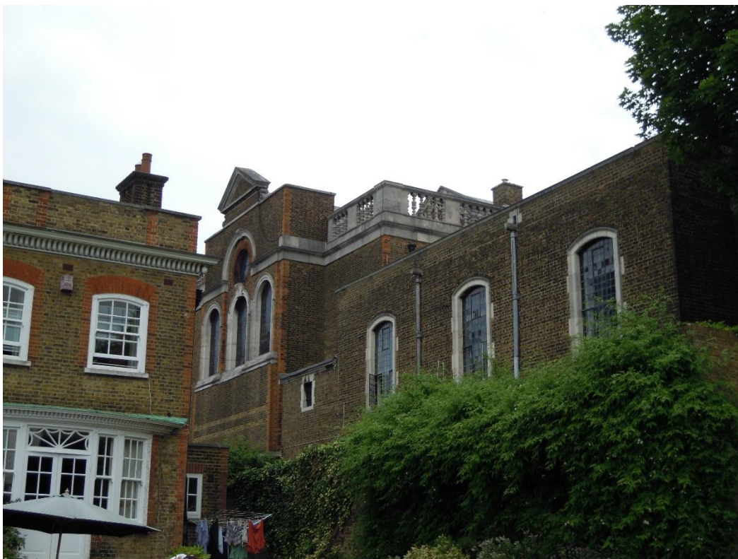
4. View of south facing chancel roof from 14 Church Row
