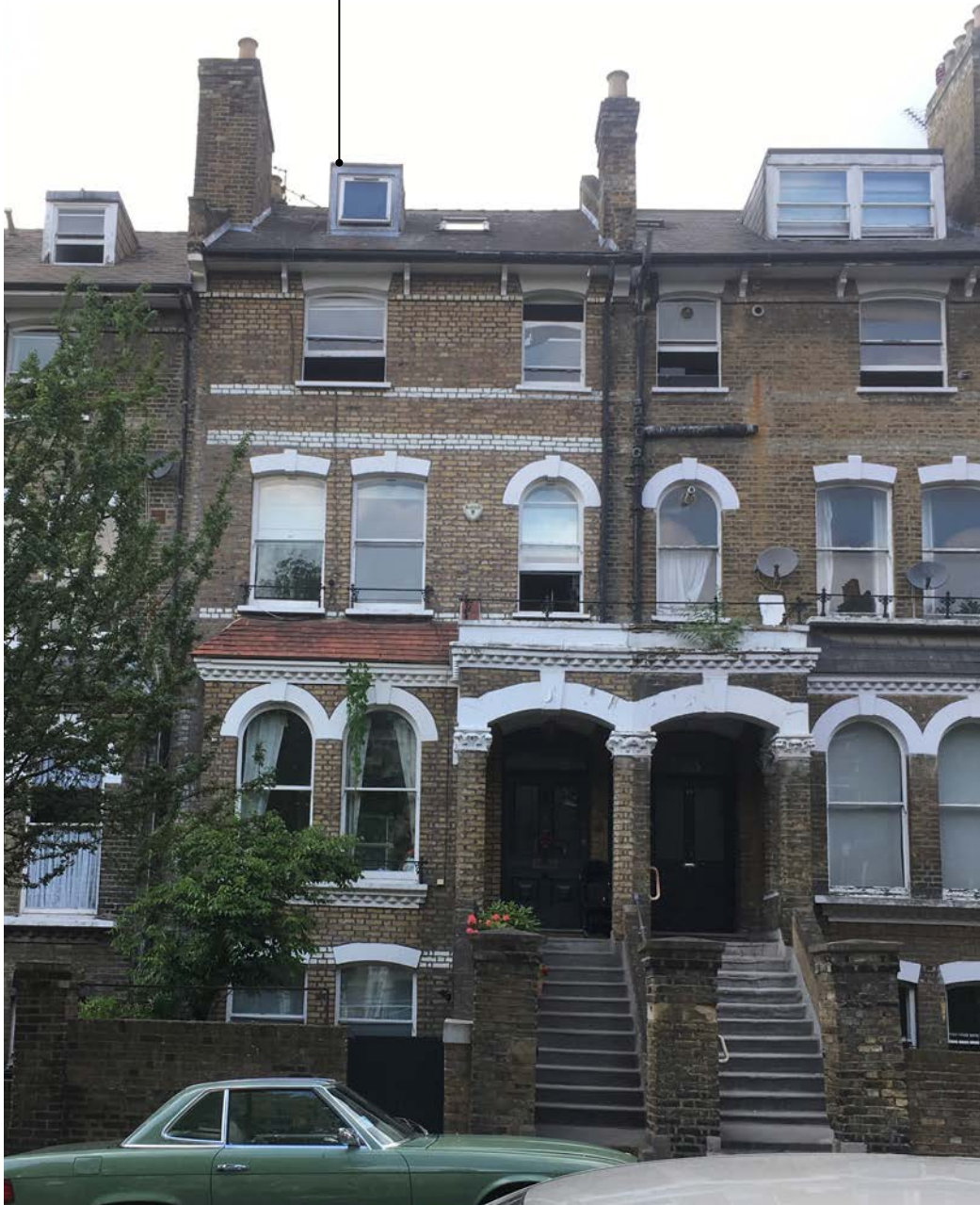
View of 81 St Augustine's Road street elevation, dormer to be enlarged.
