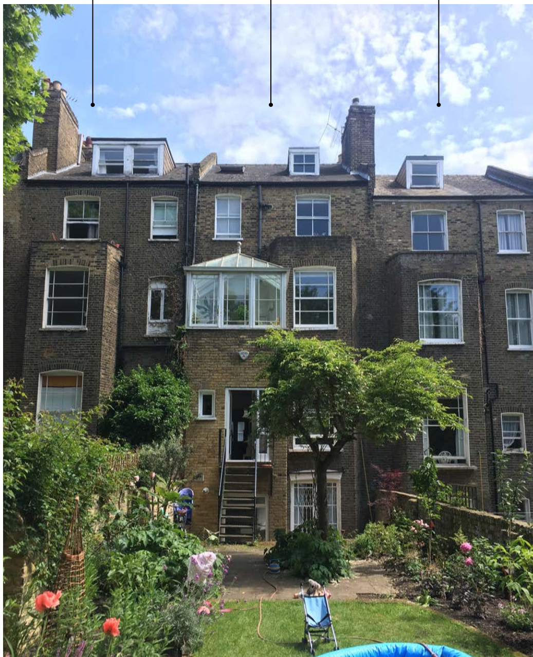
View of 81 St Augustine's Road rear elevation. Existing extension to be remodelled.
