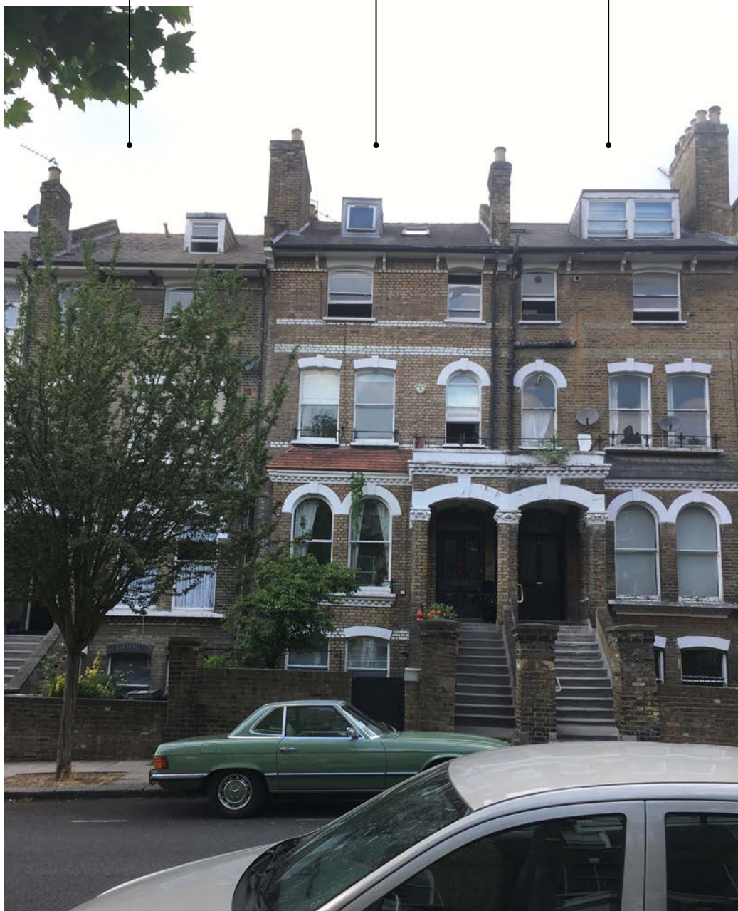
View of 81 St Augustine's Road street elevation.
