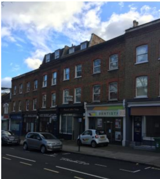
Figure 4: Example of dormer windows within the locale
