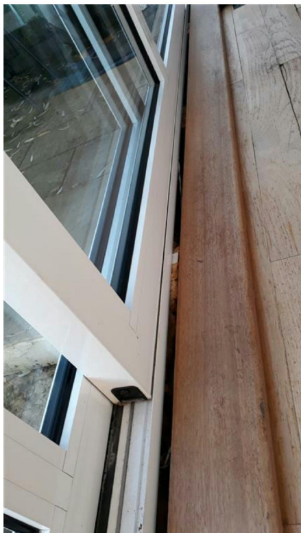
Patio doors and windows pulling away as seen by gap in floor edge
