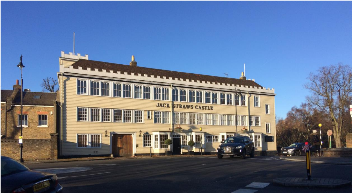
Figure 1: Front (east) elevation of Jack Straw's Castle.
