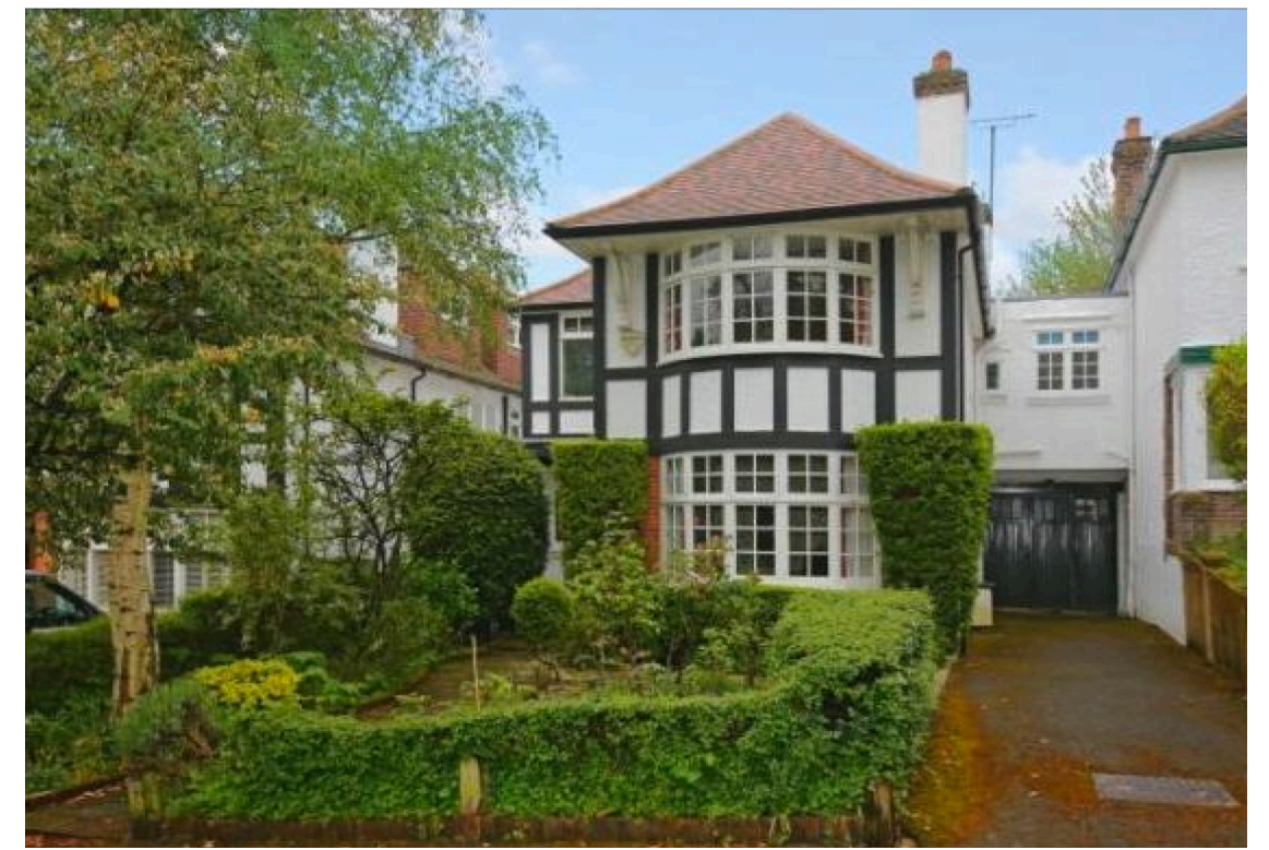
81 Hill Way - view of front elevation
