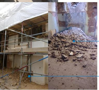
2.2 There are piles of old stone and brick loading the existing structure. Tower
