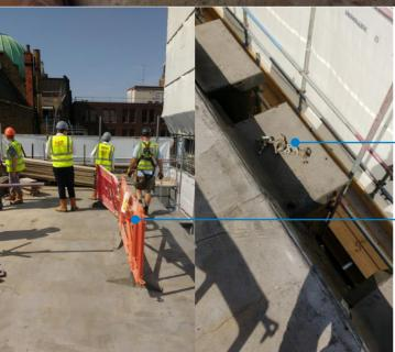
2.6 The edge protection on the roof of Bayham Place is unclear and seems to be ignored (with evidence of tools stored on a window frame below). Please ensure that a clear, safe perimeter is enforced throughout the works.
