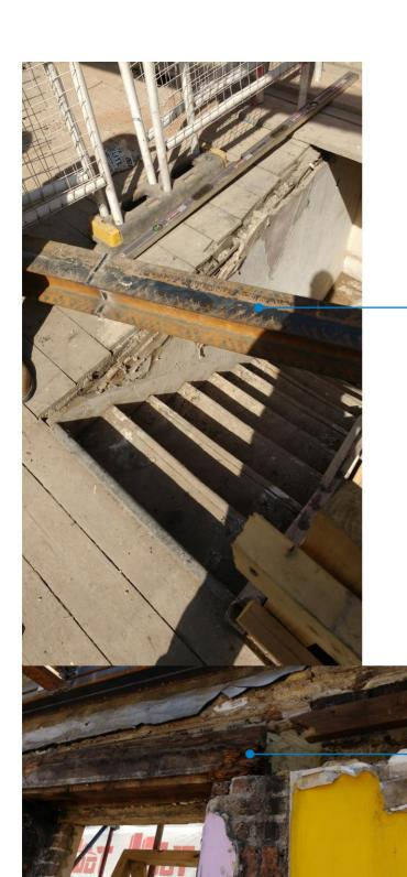
2.3 The access route to the top storey of the structure being demolished was blocked by an active flying shore. It was noted that the access would be redirected the next day. This is a H&S risk, and we ask that safe access / escape is ensured and monitored in future.
