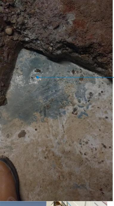
2.5 With water-ingress into thrust blocks, the concrete mix appears to have split, creating a solid,
